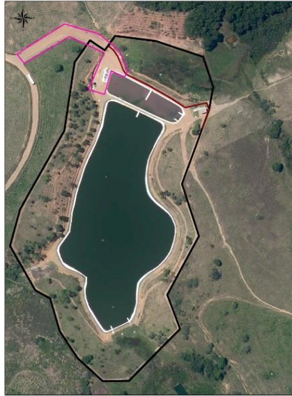
Figure 3 - Nova Rosa da Penha STP's access and sidewalk
